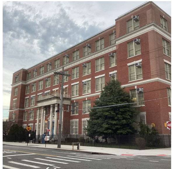
Corner of 222nd Street and 92nd Avenue - Northeast view
