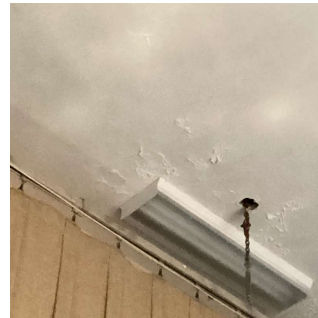
Roof 4 - Auditorium Stage
