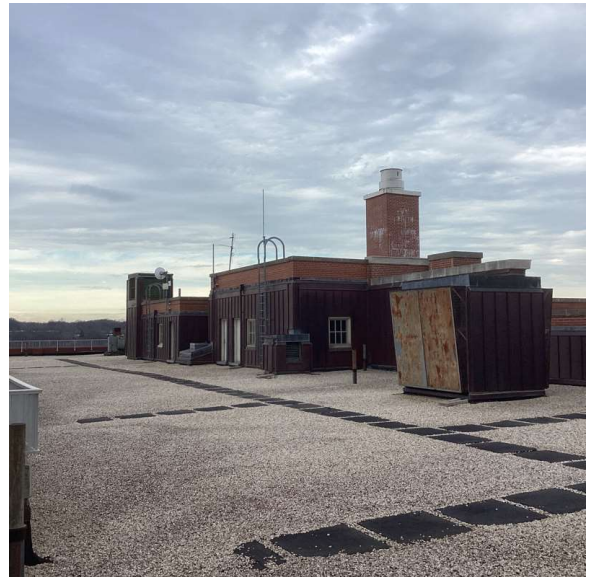
Roof 1 - Northeast view
