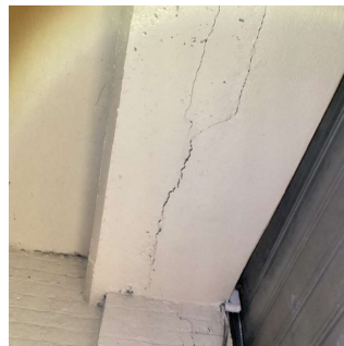
Basement - Boiler Room
