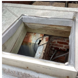
Roof 1 - Roof vent
