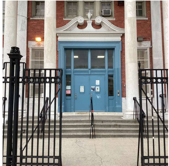
Facade A - 222nd Street
