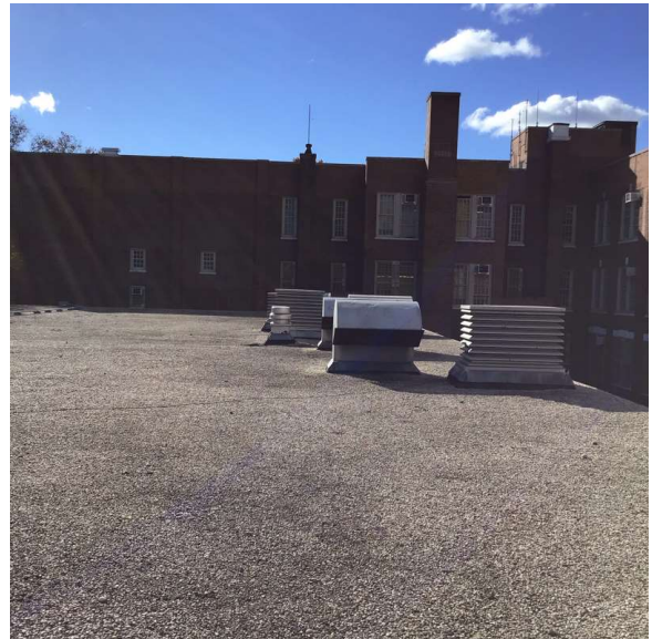
Roof 2 - South View
