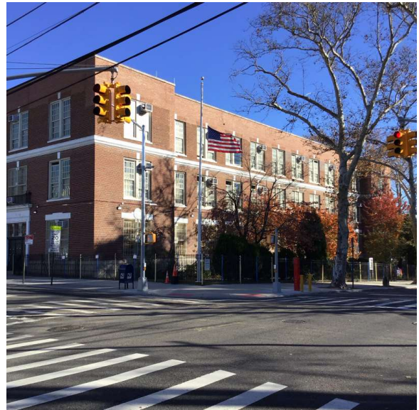
Corner of 171st Street and 35th Avenue - Northeast View
