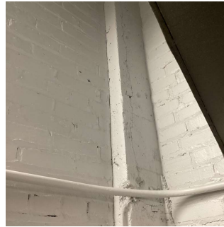
4th Floor Fan Room
