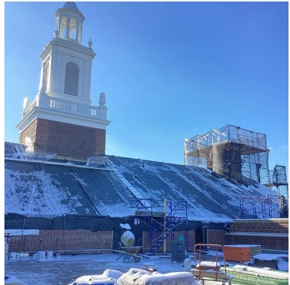
Roof 1 - South View
