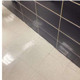
Corridor near Room 108
