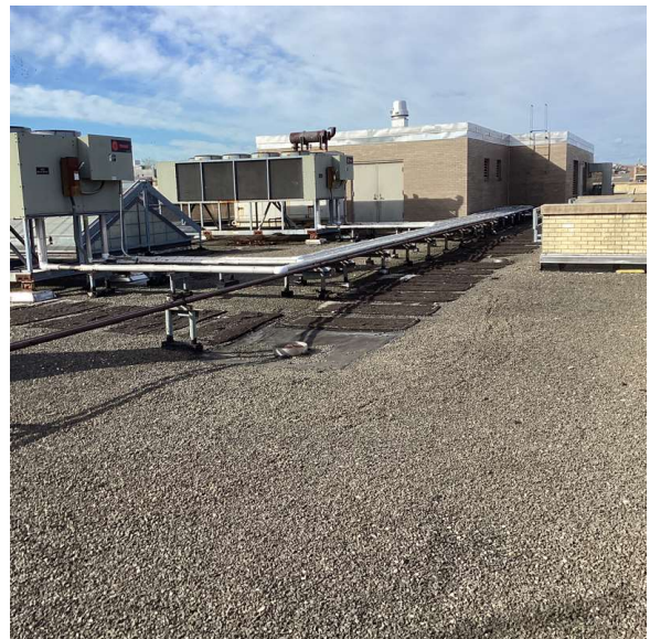
Roof 1 - Southwest View
