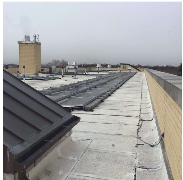
Roof 1 - Southwest View
