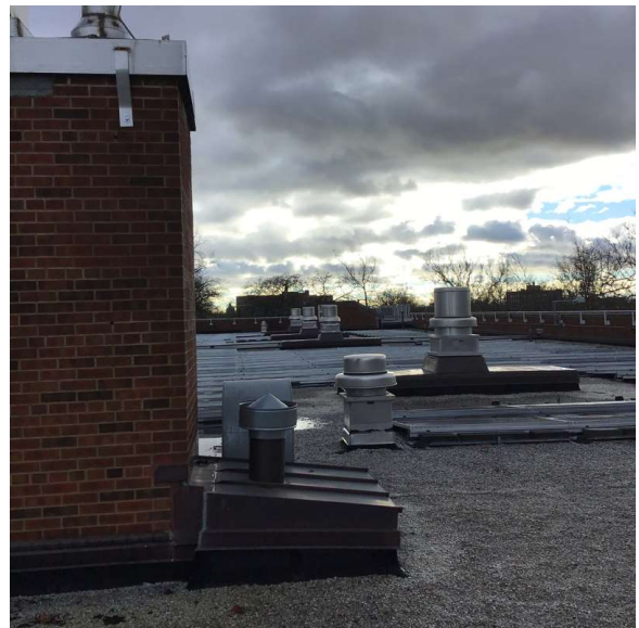
Roof 1 - South view
