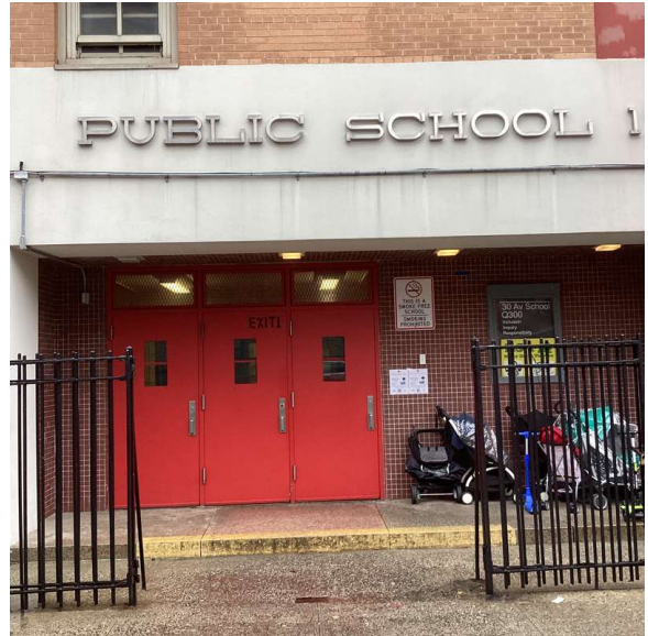
Facade A - 29th Street
