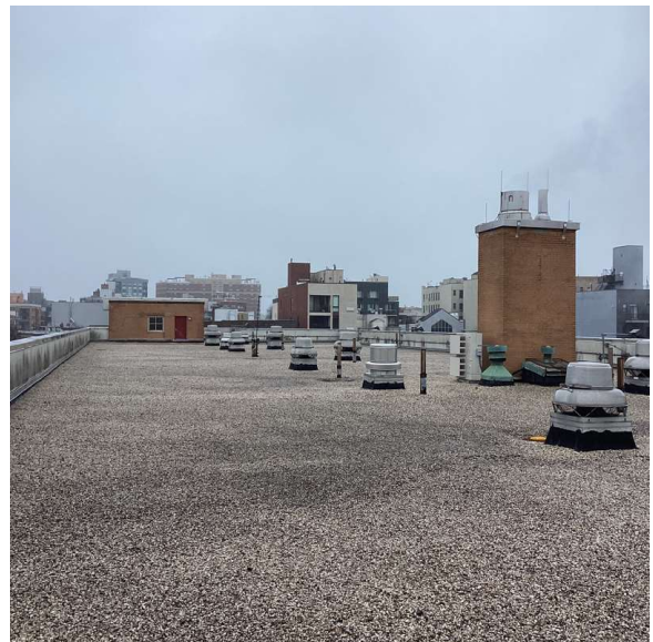
Roof 1 - Northeast view
