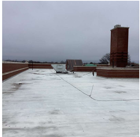
Roof 1 - Northwest View
