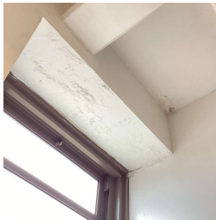
Facade A - Room 321 shown, Facade A - Room 317 similar
