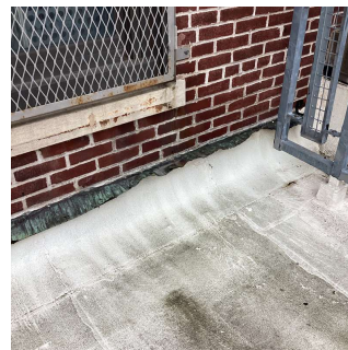
Roof 5 - Facade E
