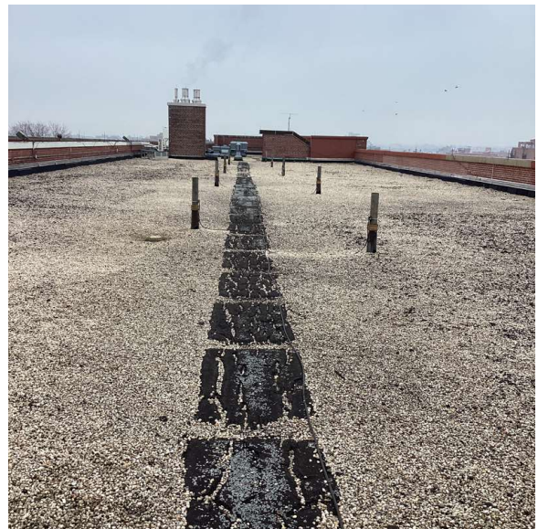
Roof 1 - Southeast View
