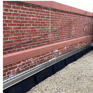
Roof 1 - Facade A
