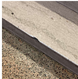
Main Entrance Lobby
