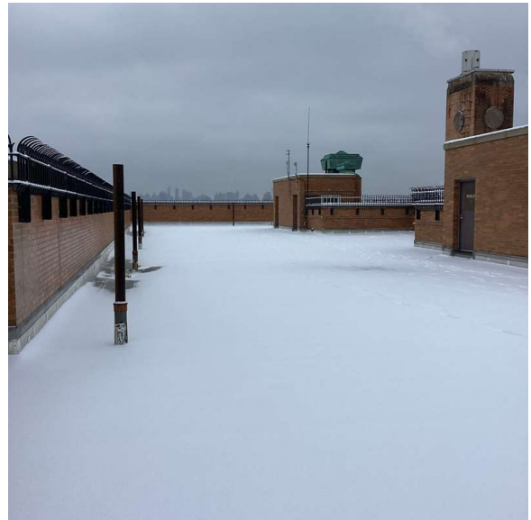
Roof 1 - Northwest View
