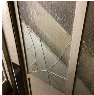
Stair E/F Bulkhead
