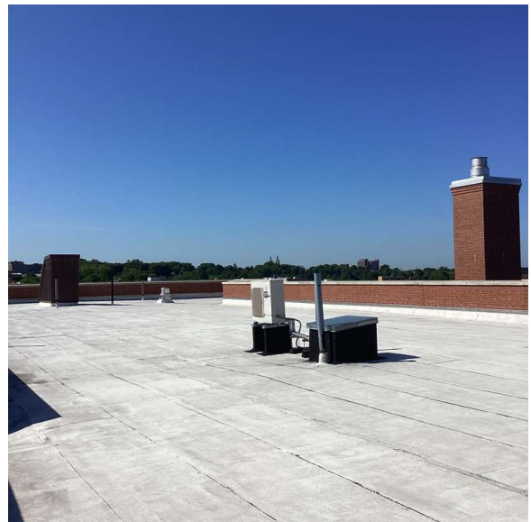
Roof 1 - South view
