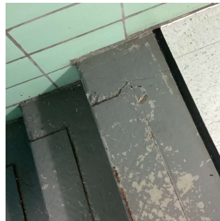
Corridor near Room B44
