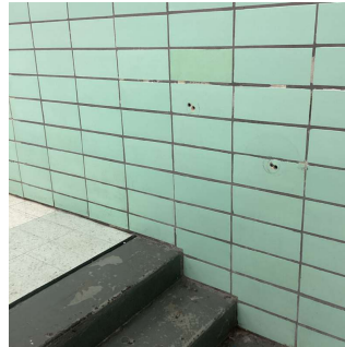
Corridor near Room B37
