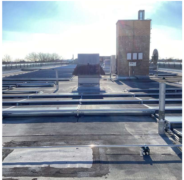
Roof 1 - Southeast view
