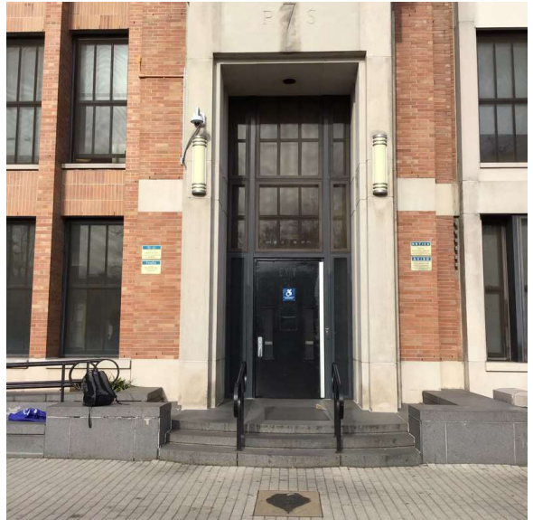
Facade A - Cornice Avenue
