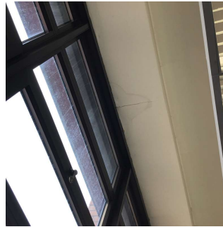
Corridor between Auditorium and Gymnasium
