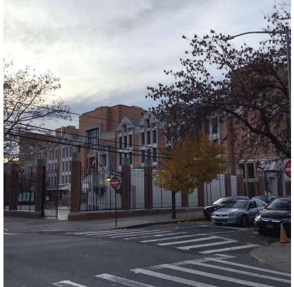
Corner of Poyer Street and Cornish Avenue - East View
