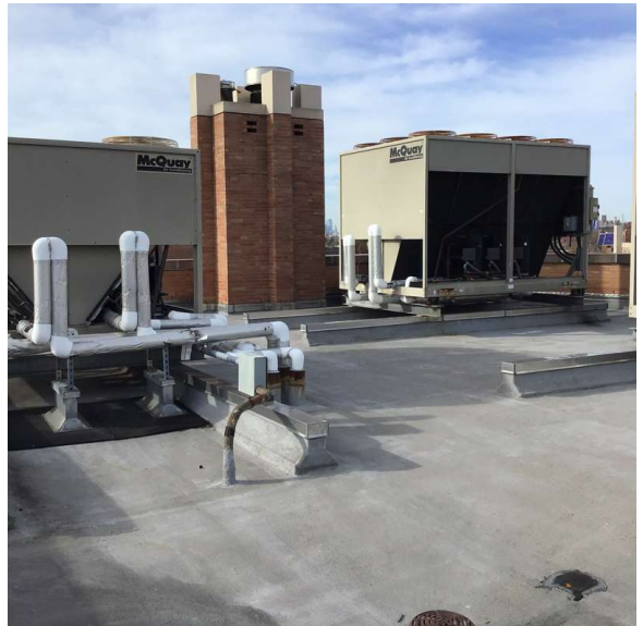
Roof 1 - East View
