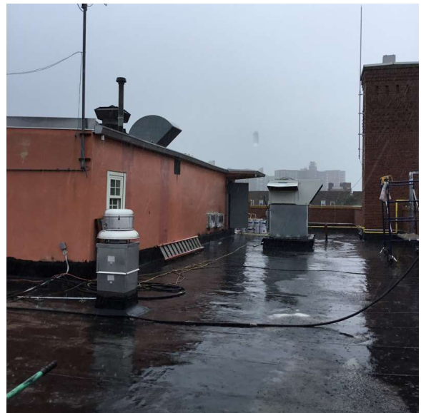
Roof 1 - West View
