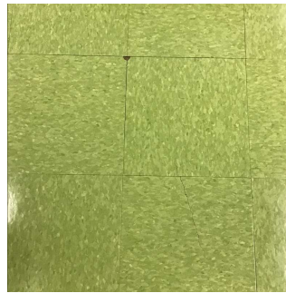
Corridor near Room 305
