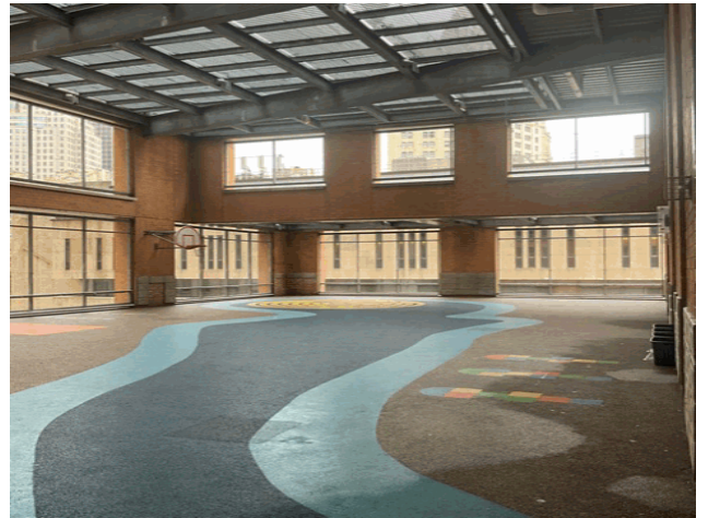
Roof 1 (Plaza Deck) - Northwest View
