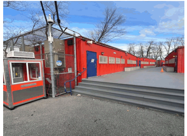
TCU T30 - North View
