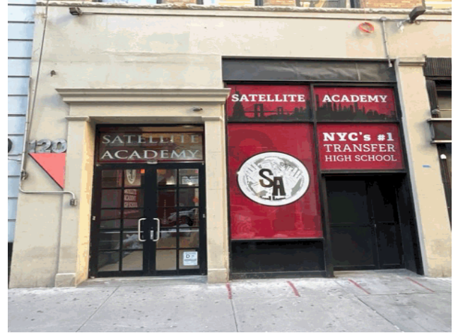
Facade A - West 30th Street
