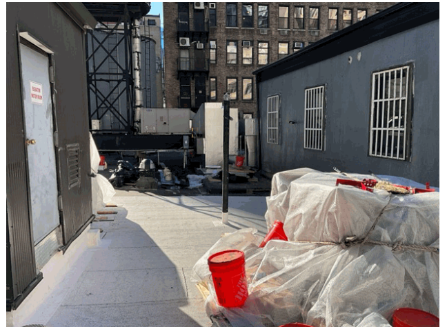
Roof 1 - South View
