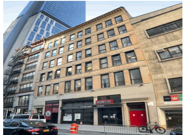
West 30th Street - South View
