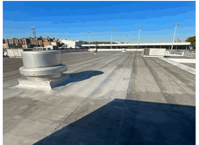
Roof 1 - Northwest View
