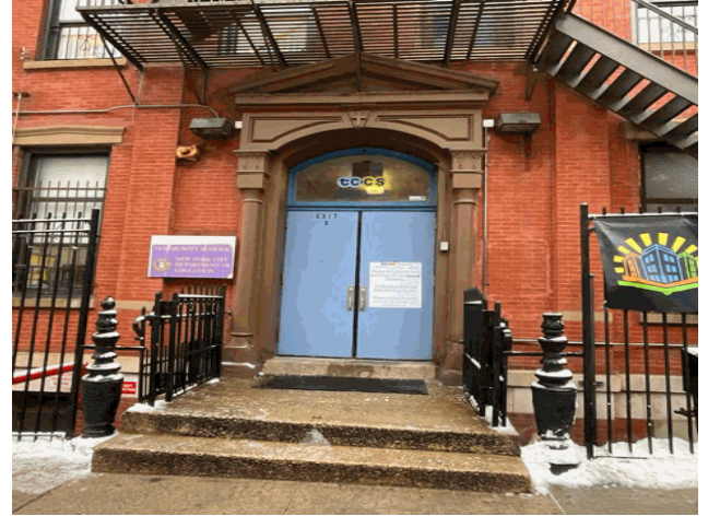
Facade A - Morningside Avenue
