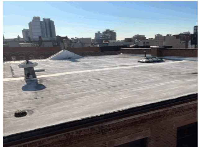
Roof 1 - Southeast View
