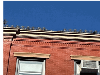
Roof 1 at Facade A
