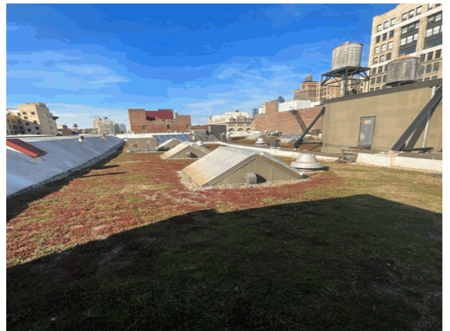
Roof 2 - Northwest View
