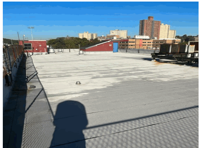
Roof 1 - Northwest View
