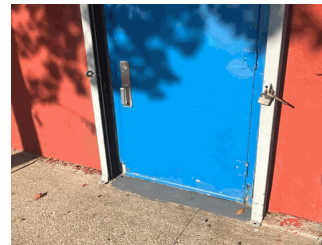
Boiler Room Door
