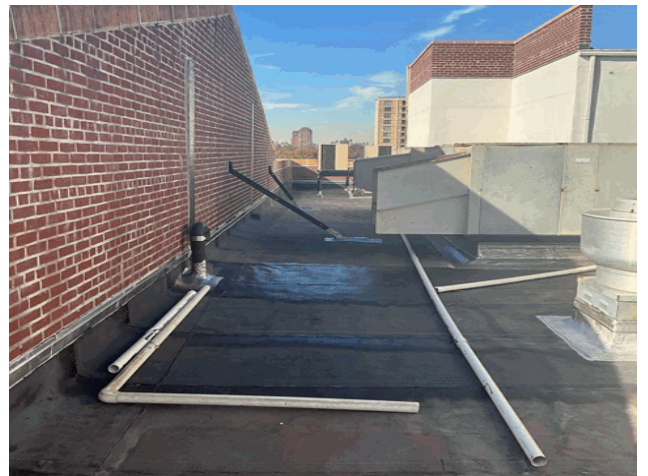
Roof 1 - West View
