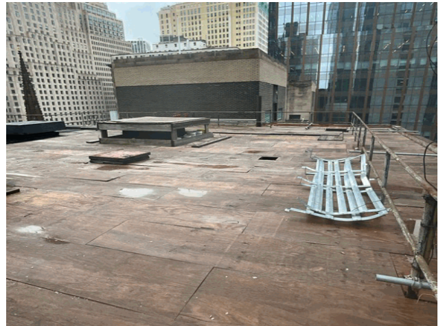
Roof 1 - South View
