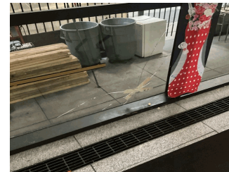
Facade D - 1st Floor Lobby
