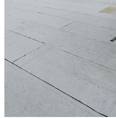
Roof 1 - North View
