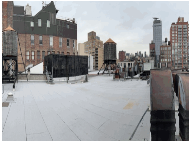
Roof 1 - North View
