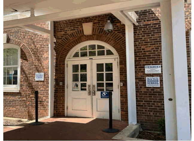
Facade A - Wheeler Avenue
