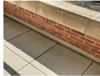
Facade A on Plaza Deck
