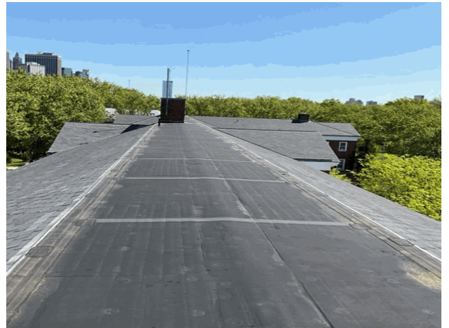
Roof 1 - Northeast View
