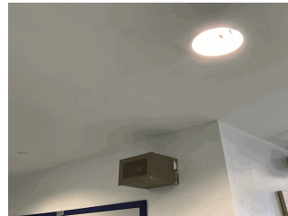
Corridor near Room 300.2
