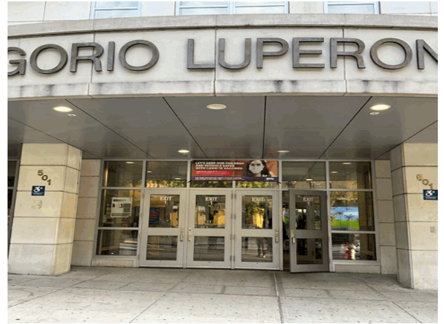
Facade A - West 165th Street
