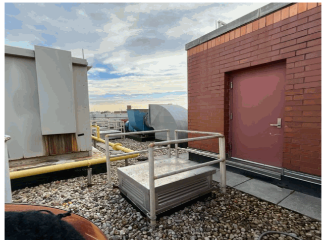
Roof 4 - Northeast View
