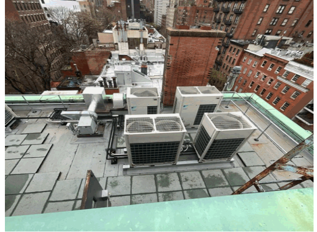
Roof 1 - Northwest View
