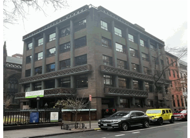
Corner of West 12th Street and 5th Avenue - West View
