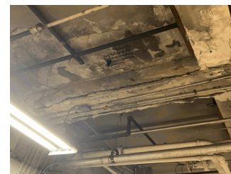
Storage Room below Lobby shown, also in Room 312
