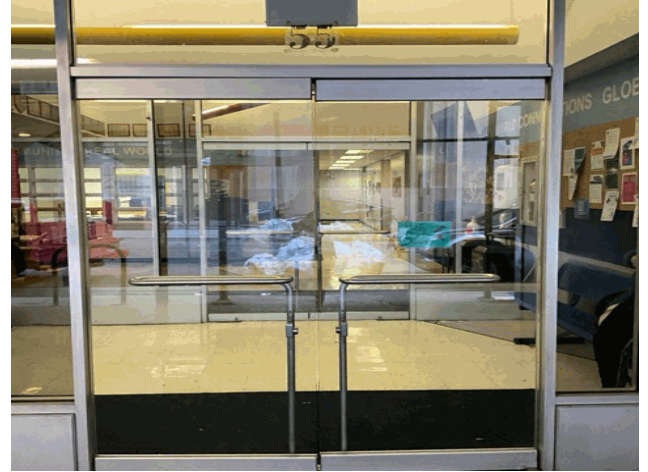
Facade A - East 25th Street
