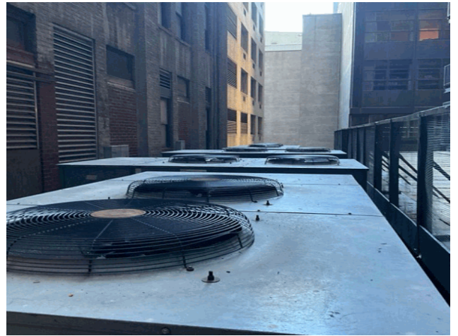
Roof 1 - Northwest View
