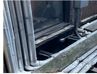
Facade C at Roof 1
