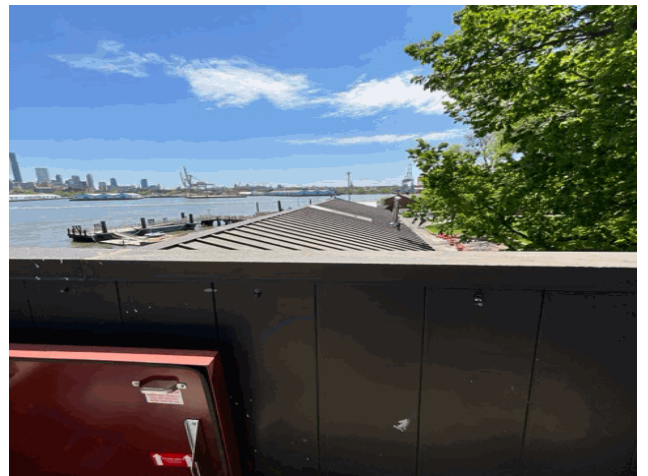
Roof 1 - Southeast View
