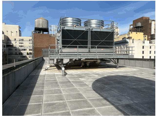
Roof 1 - Northwest View
