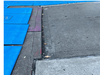
Bottom of Ramp at Exit 3
