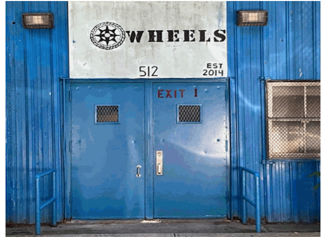
Facade A - West 182nd Street
