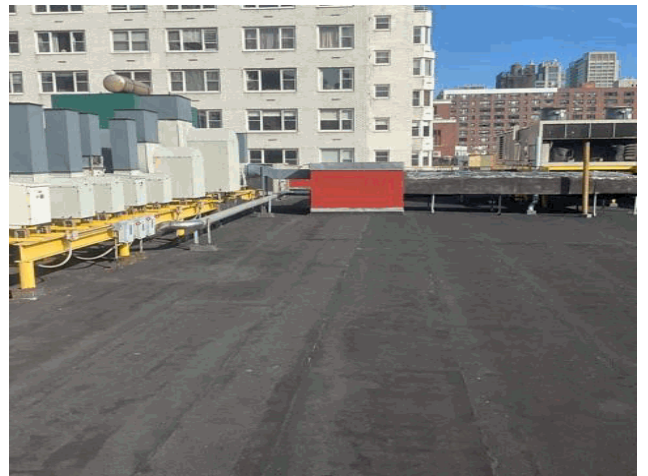
Roof 1 - North View
