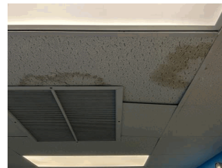
Corridor near Room 102 shown, also Room 105A
