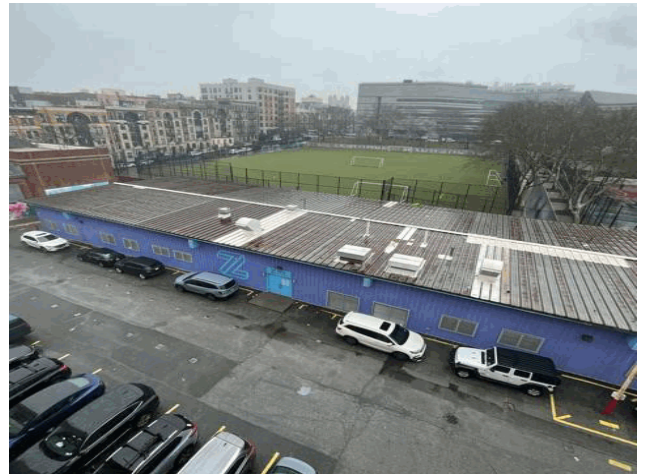
Roof 1 - East View
