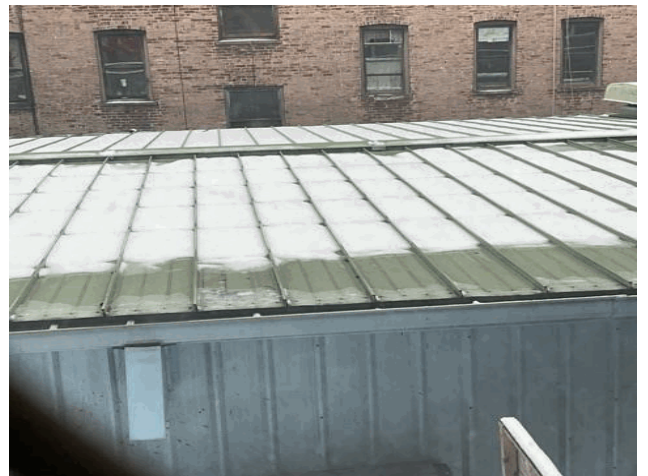
Roof 1 - West View
