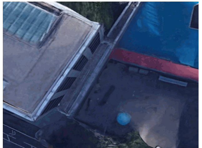
Roof 1 - Aerial View
