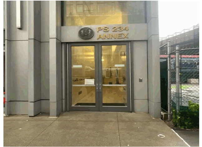
Facade A - Warren Street
