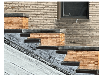
Facade B at Roof 3
