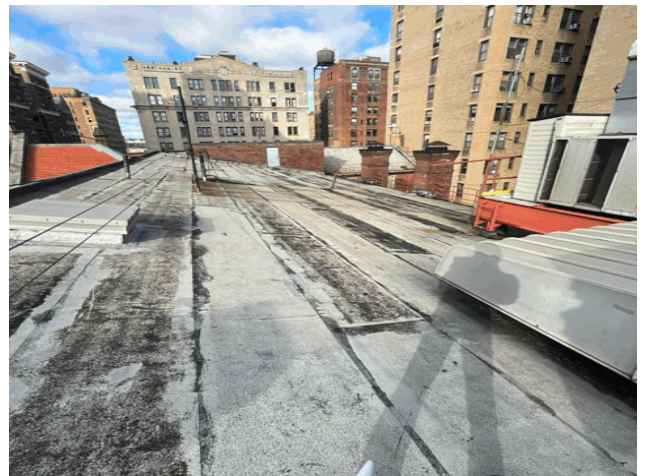
Roof 2 - Northwest View
