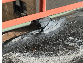
Roof 4 at Facade D
