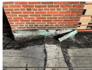
Roof 4 at Chimney CH2
