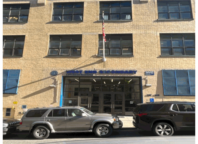
Facade A - 61st Street
