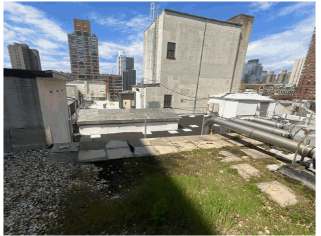
Roof 4 - West View
