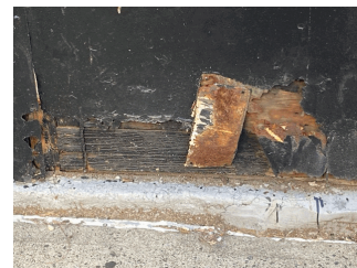
Access door to 55th Street Electrical Room
