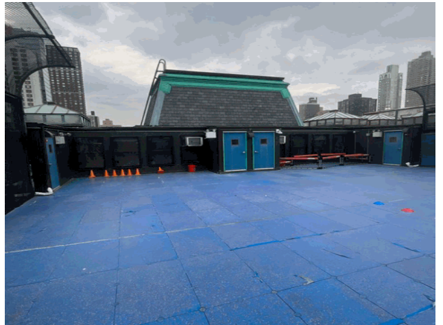
Roof 1 - Southwest View
