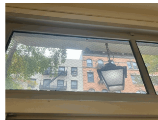
Facade A - MPR Entrance
