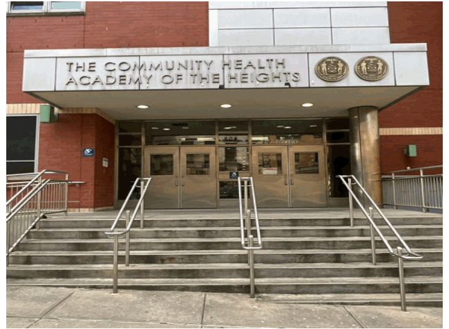
Facade A - West 158th Street
