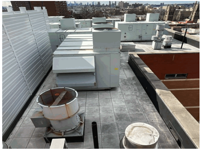
Roof 1 - Southwest View
