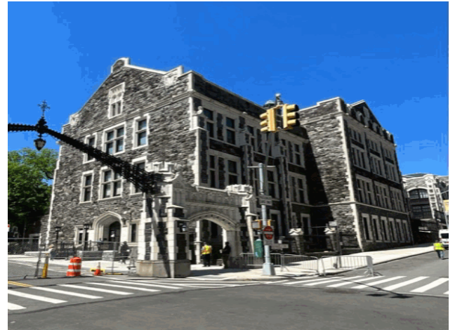
Convent Avenue and West 140th Street - West View
