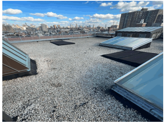
Roof 1 - Northeast View
