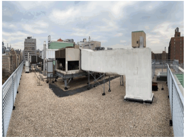
Roof 1 - North View
