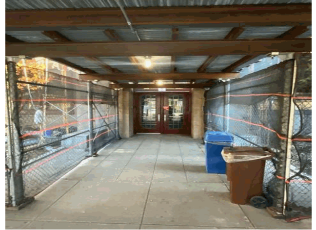
Facade A - East 96th Street
