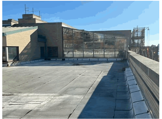
Roof 3 - East View
