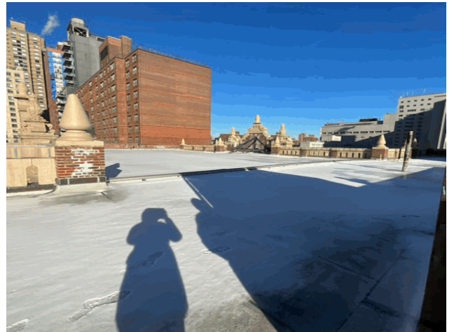
Roof 1 - Northwest View
