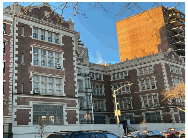
East 96th Street - Northwest View
