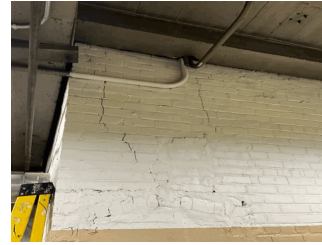
Chimney (in Boiler Room)
