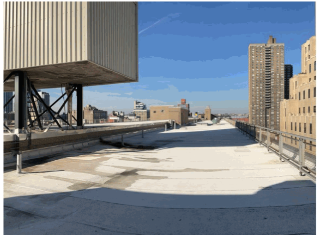
Roof 1 - Northwest View
