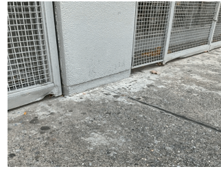
Facade A (at Exit 6)
