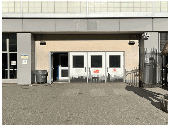
Facade A - West 49th Street
