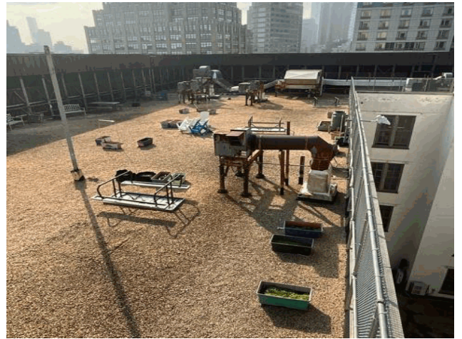
Roof 1 - South View
