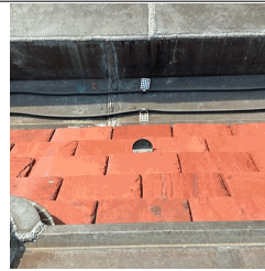
Roof 3 - Facade C
