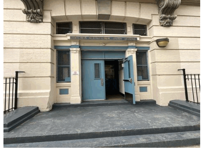
Facade A - Dominick Street
