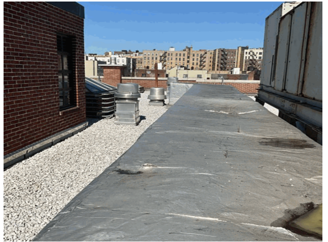
Roof 1 - West View
