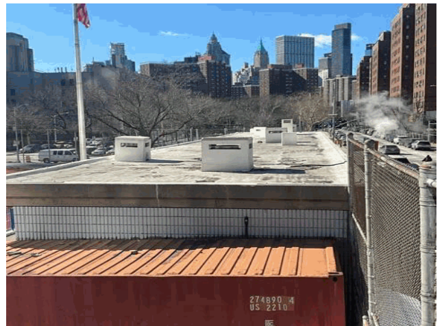
Roof 1 - West View
