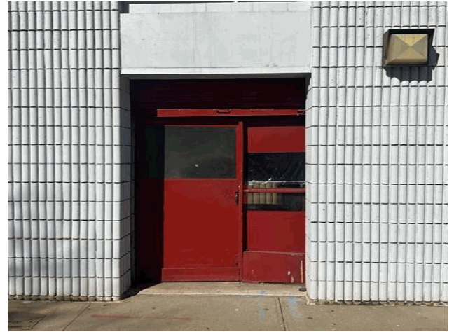
Facade A - North View
