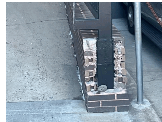
Exit 7 - Service Ramp
